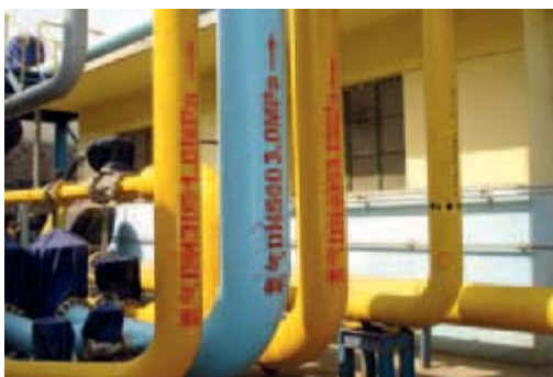
Carrying out anti-corrosion works
