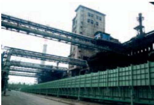
Construction of a machine-side furnace head smoke ground dust removal station
