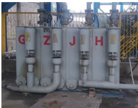
Replaced with anti-gas leak drainer
