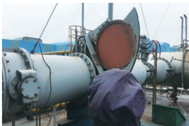
All gas pipelines with a diameter of less than 1.8 meters were upgraded to be equipped with electric blind flange valves
