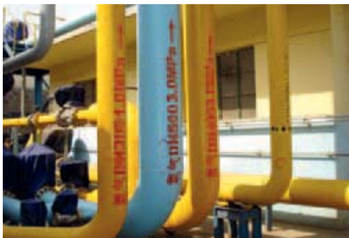
Carrying out anti-corrosion works
