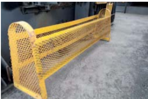
Mechanic guarding rectification
