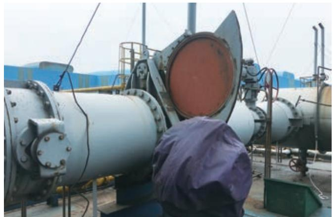
All gas pipelines with a diameter of less than 1.8 meters were upgraded to be equipped with electric blind flange valves
